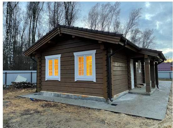
A completed house, finished and painted
