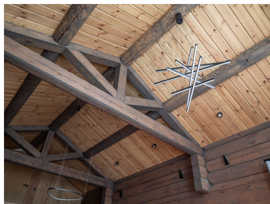
Exposed roof structure over a finished room
