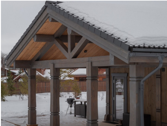
Carved-post veranda, completed
